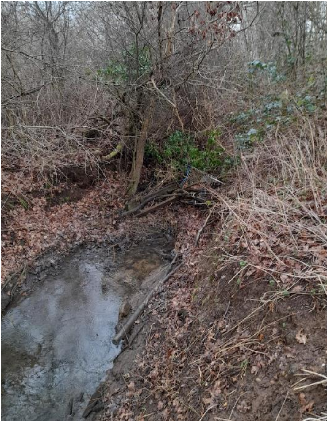
Photo 5. General vegetation blockage in the ditch. The direction of water flow is from the bottom left towards the centre of the photograph. -----
