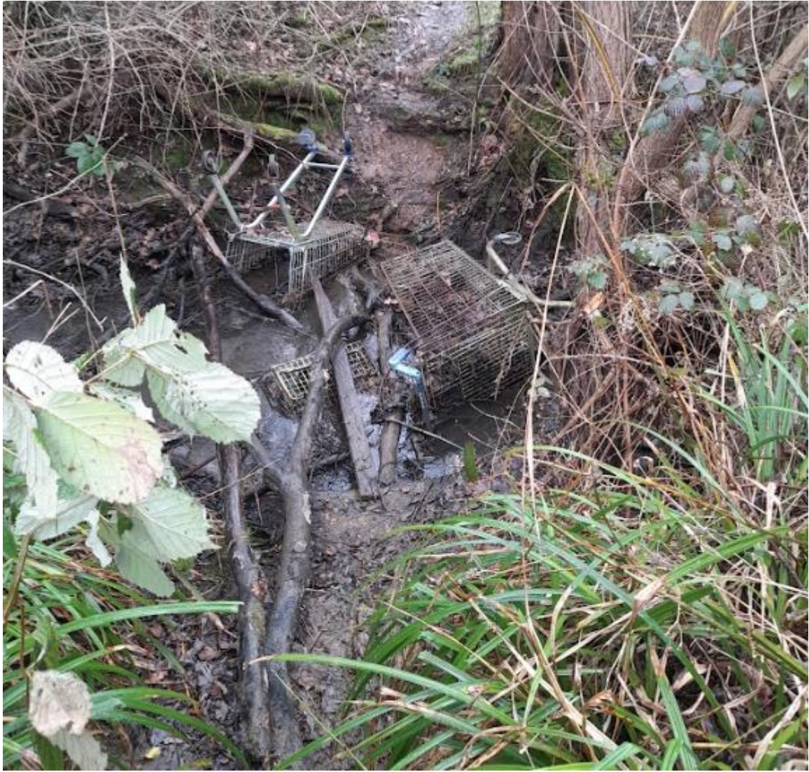
Photo 2. An ad-hoc crossing point from land owned by Central Bedfordshire Council created in the drainage ditch, resulting in partial blockage. The direction of water flow is from left to right.
