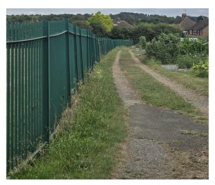
Officers instructed a contractor to have a look and quote for the repair of the fence. It was reported back that the footings were not deep enough and lack concrete. Therefore, the fencing would continue to lean and progressively get worse if it is not repaired. The fencing was originally installed some time ago and so it would not be covered under any warranty. The section of fencing requiring repair measures 130m and the whole section would need repairing.
