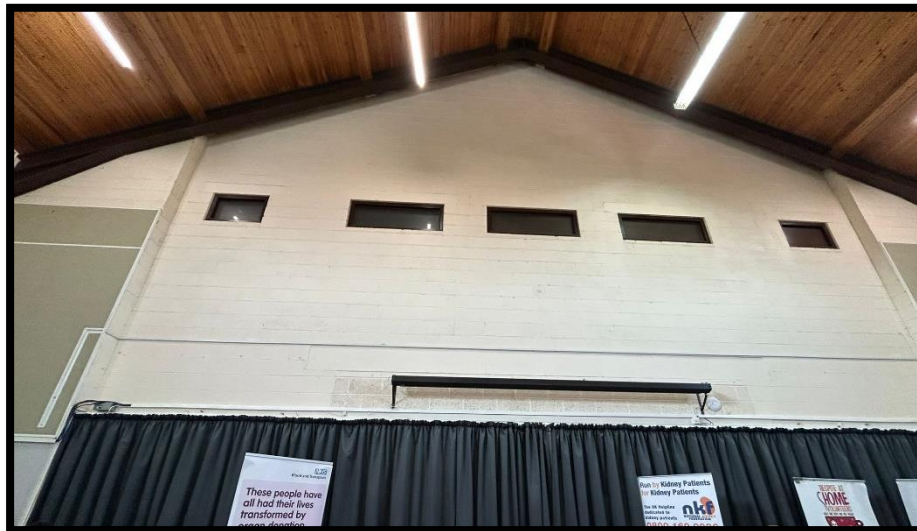
Figure 2 - Gable end wall (blockwork)
