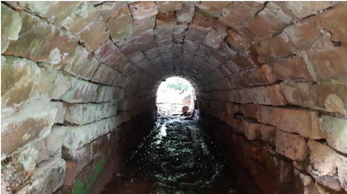
Fig 15 - The brick vaulted culvert
