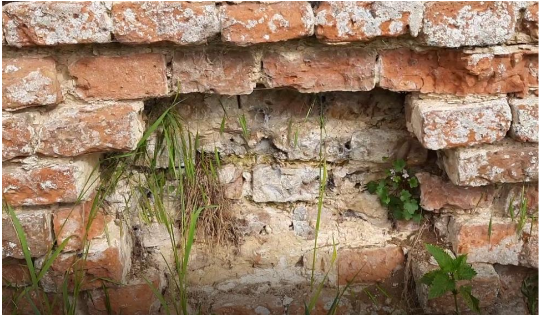
Fig 04 - Ha-Ha, showing a cavity which is half a brick width deep
