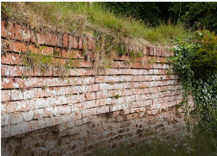
Fig 05 - Ha-Ha, showing cavities and open joints
