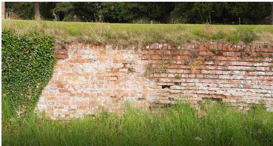
Fig 03 - Ha-Ha, showing section that has been rebuilt/consolidated
